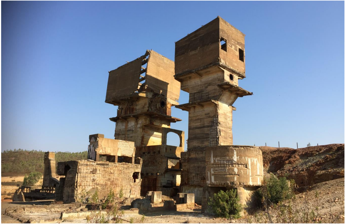
This structure is located at the location marked White-Rumped Swift on the map below..
