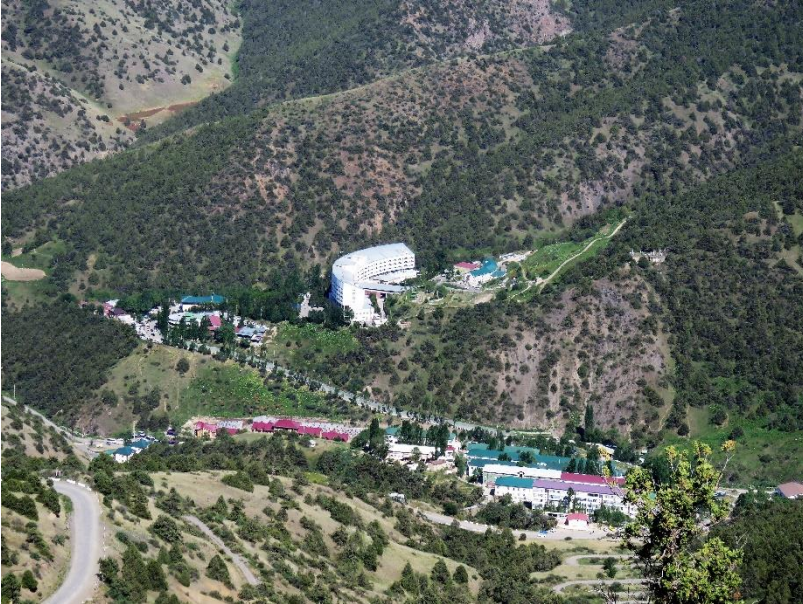
An overview of the sanatorium and the path to follow on the ridge over it
